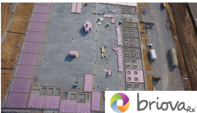
Pink Thermo Mass Insulated Wall Panel Installation
