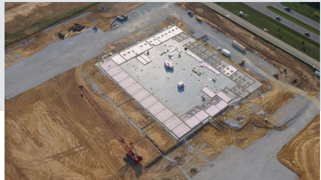
Concrete Cast-in-Place Wall Panel Fabrication on Floor Slab
