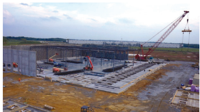
Concrete Tilt Wall Panel and Steel Erection Southwest
